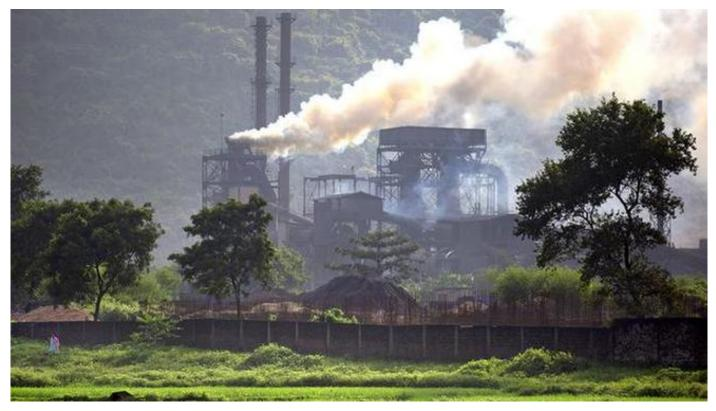
Thermal power plants generate roughly 70% of India's electricity by burning coal, which also releases some sulphur that can go on to form highly reflective sulphate aerosols. | Photo Credit: Altaf Qadri
